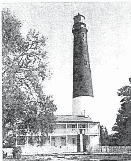
The Keepers' Dwelling and the tower.
