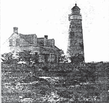
Key West Lighthouse prior to 1886, showing the original dwelling which was pre-fabricated and brought down to Key West on the lightship Honey.
