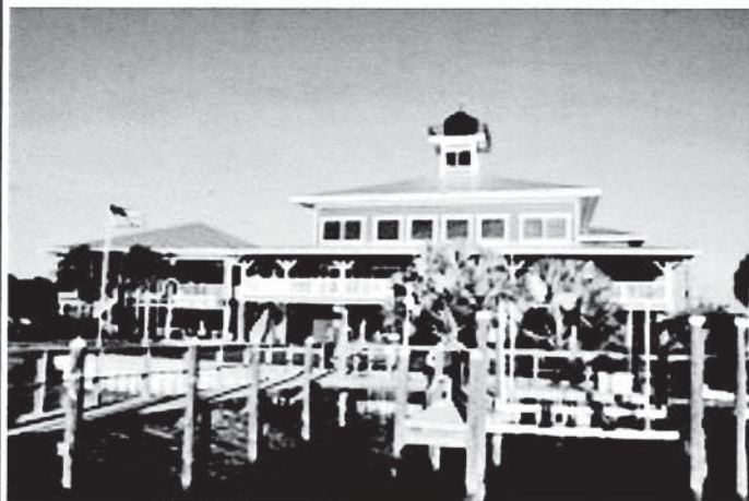
Left, Tampa Bay Watch facility. Note, the top is a Coast Guard recognized lighthouse.
